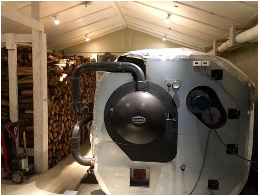
The boiler is draft induced with a blower, thus air is pulled through two combustion air dampers. The primary air damper controls the flow to the base of the batch of wood, manipulating the amount of wood gas produced. The secondary air damper supplies pre-heated fresh air to the insulated secondary burn chamber where it meets the wood gas. This mixture re-ignites on average to 1800°F, consuming most volatiles. This superheated, clean flue gas with a
